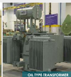
OIL TYPE TRANSFORMER
