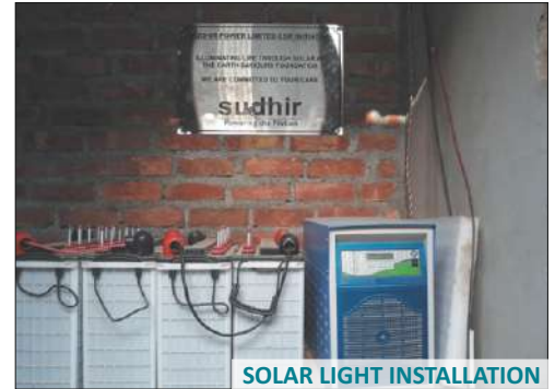
SOLAR LIGHT INSTALLATION
